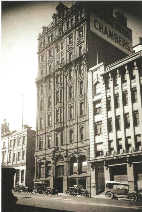
IOA Office Melbourne (on right) 1924 54 - 56 Market St, Melbourne
